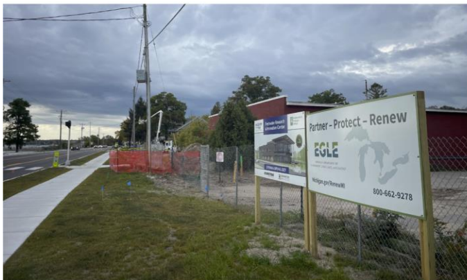
Construction site for the Freshwater Research and Innovation Center
